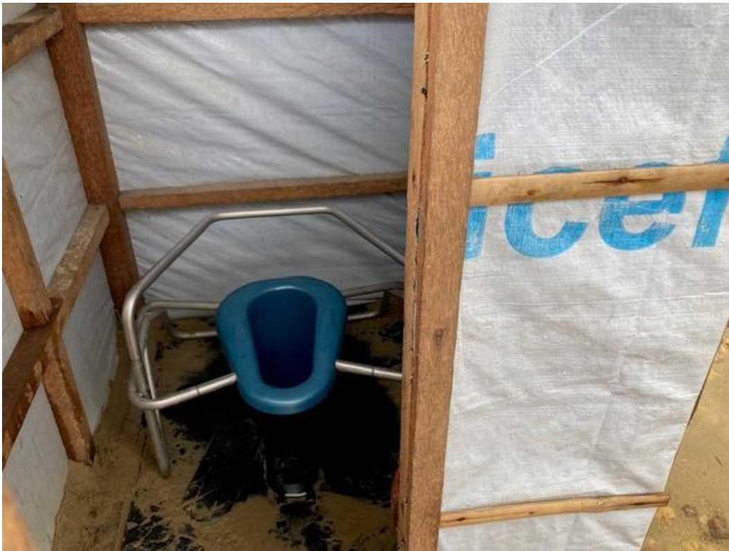
One of the community toilets in Roxas, Palawan, has raised toilet seats, safety frames, and rails that improve toilet accessibility for the elderly and people with disabilities. (Photo credit: UNICEF/PHL/Vasquez)
